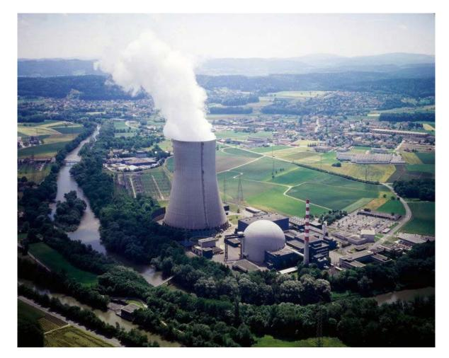
PWR type (Siemens) 3-loop plant since 1979 in operation
