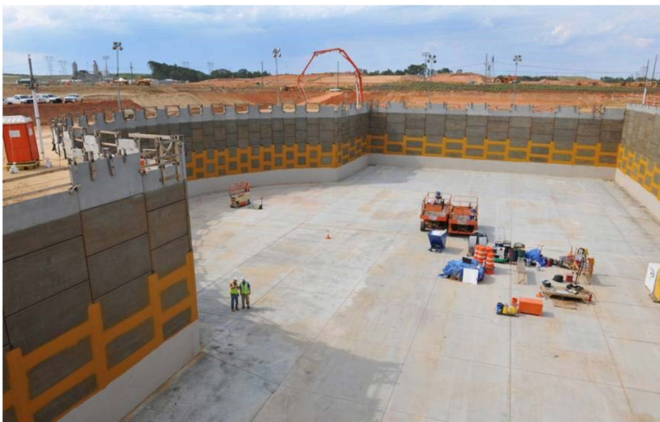
Vogtle Unit 3 "nuclear island," with water proofing work in progress; location where containment vessel and associated nuclear components will be placed.
