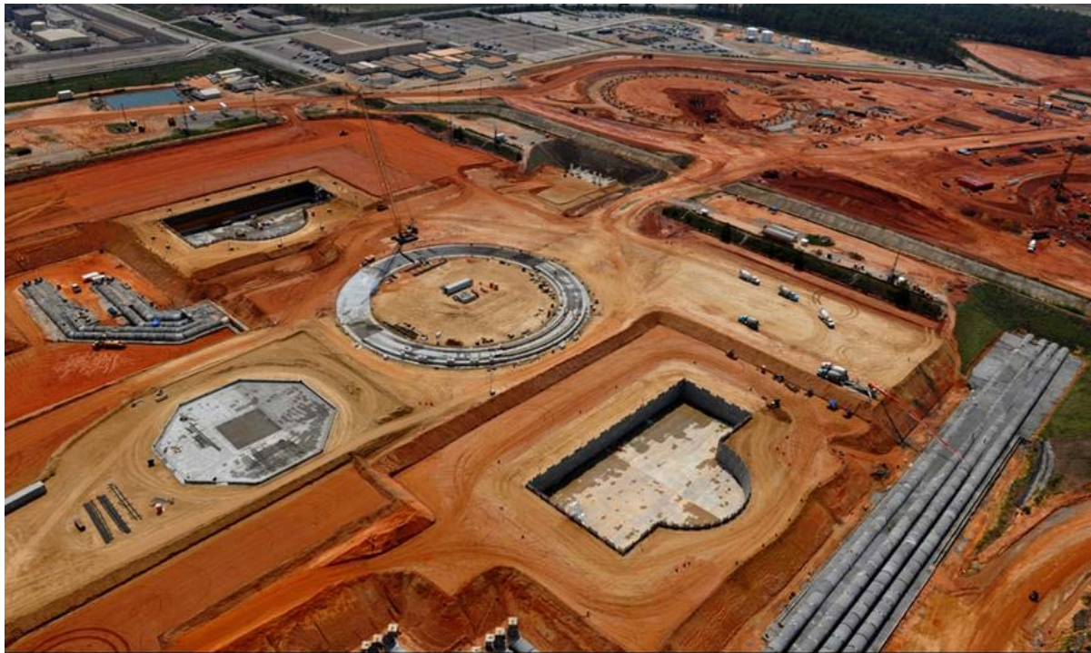
Aerial photograph of Vogtle 3 and 4 construction site. Unit 3 is located at left and top of photo and Unit 4 to the right and bottom. Heavy lift derrick crane foundation in center.
