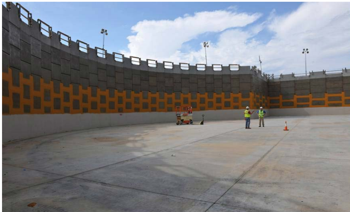
Vogtle Unit 3 "nuclear island," with water proofing work in progress; location where containment vessel and associated nuclear components will be placed.
