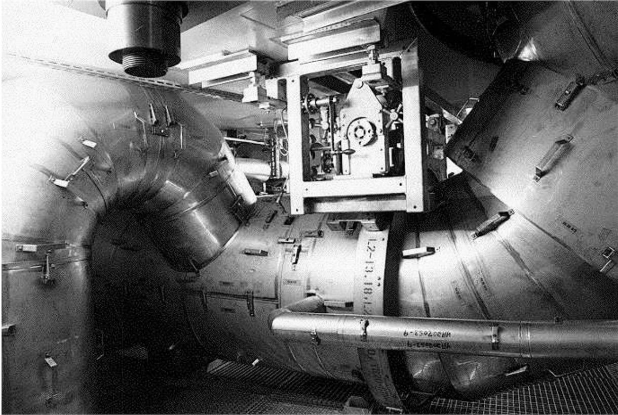
Figure 4: Main coolant pipe inspection rails
