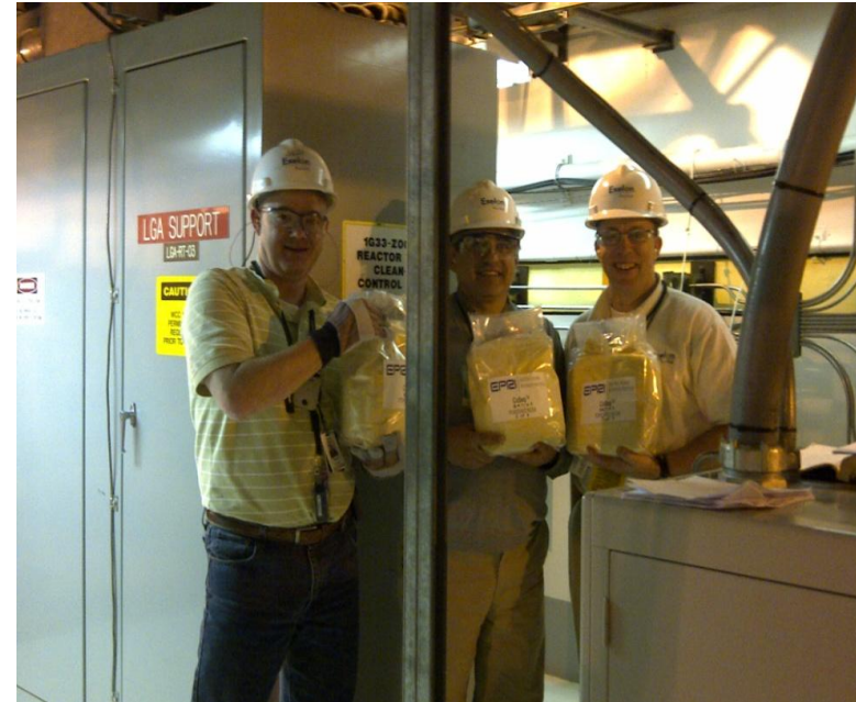
EPRI Resin Loading into LaSalle Reactor Water Cleanup System for Demonstration Tests - April 2012
