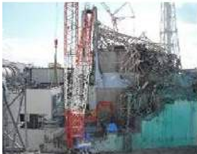
Damaged by Hydrogen Explosion As of Feb. 12, 2012
