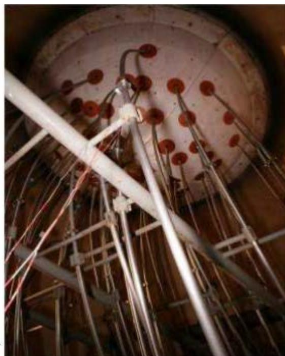
Figure 3: Guide tubes in the reactor pit
