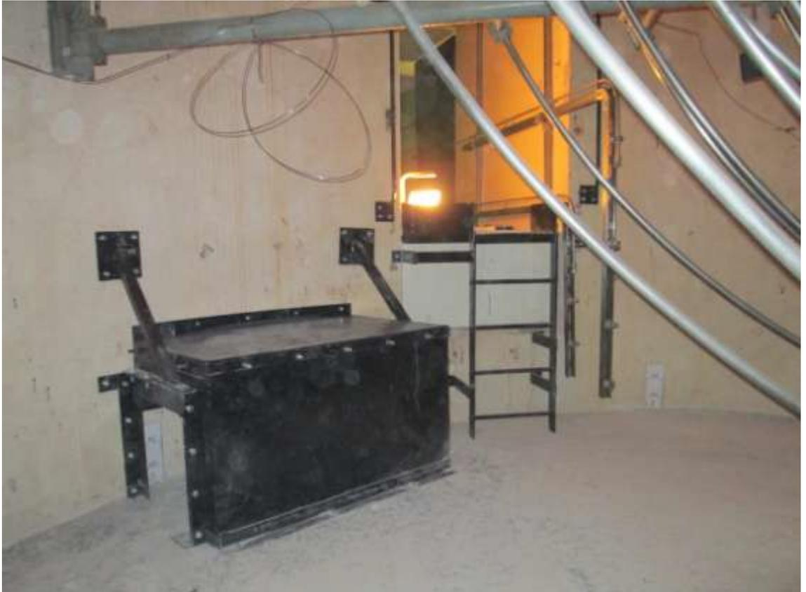
**Figure 12: Biological shield in the reactor pit**
