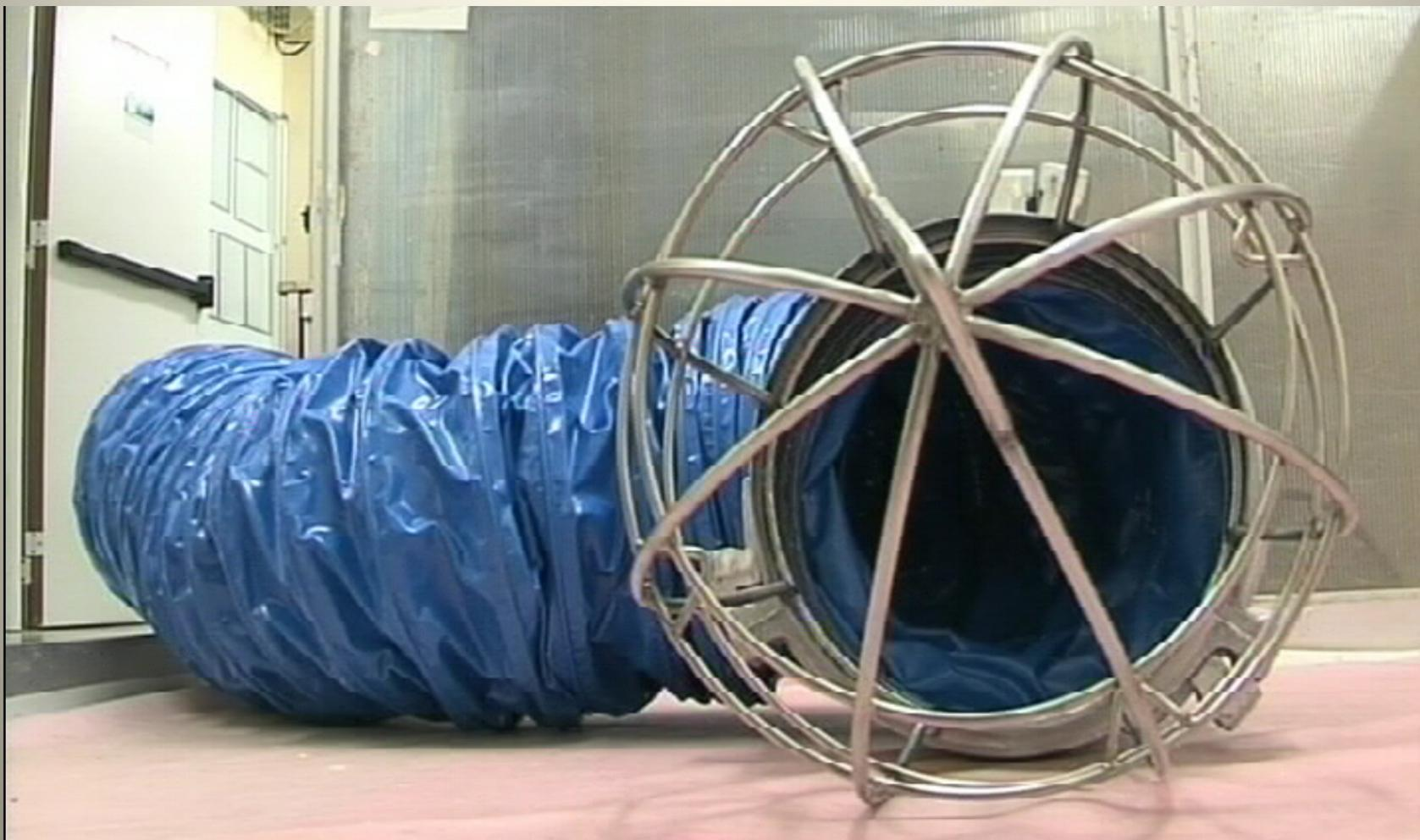
The sphere cage can be adapted to different duct diameters. The ZAG couplings will then be used for DN 300, 200, 170 or 150.
