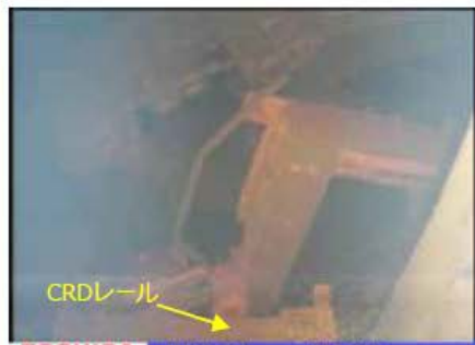
CRD Exchange Guide Rail
