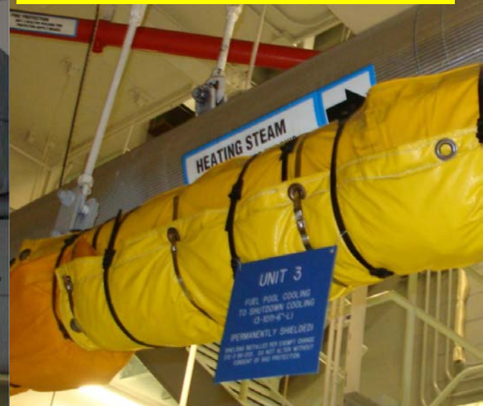
Steam pipe heater to protect frozen
