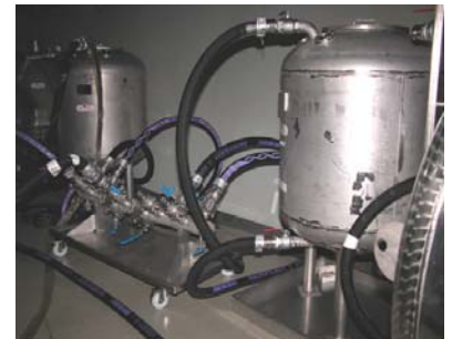
Emmac chemical process
