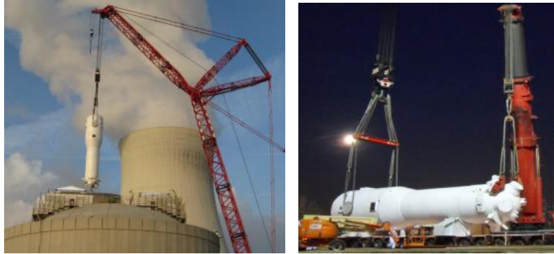
Figure 2 - Overview of the lifting operation of the old steam generators.
