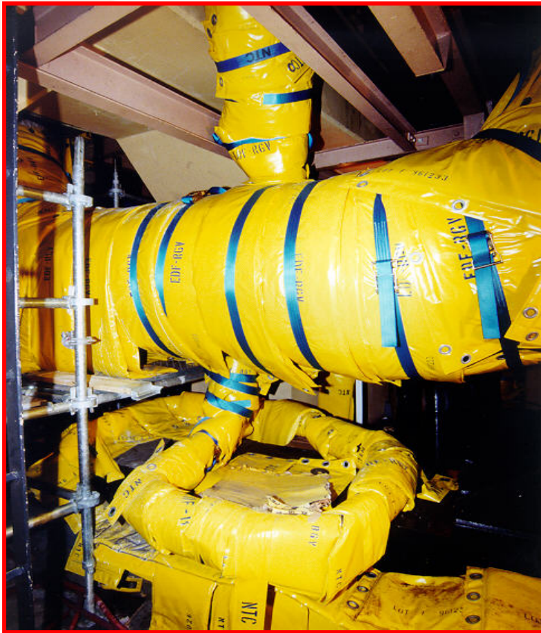
Biological Shielding strapped on the piping
