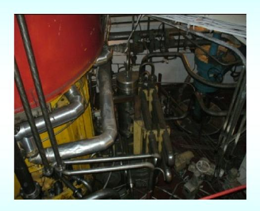
1. Decrease of gamma dose rate from sealing water pipes (presence of high radioactive point sources in the pipes gave dose rate around 10-100 mSv/h).
