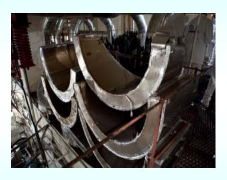
An example of steam generator quick detachable thermal insulation cassettes
