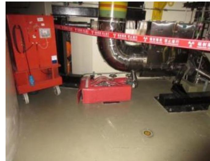
Hot Spots Shielding And Removing—6. Flushing of chemical sampling pipeline
