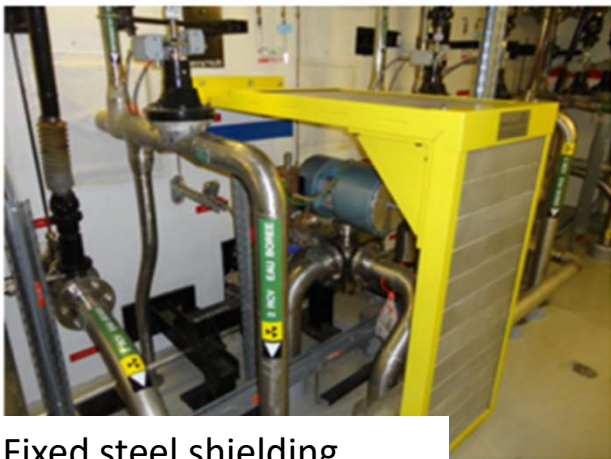
Fixed steel shielding
