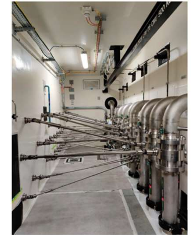
Valve remote controls
