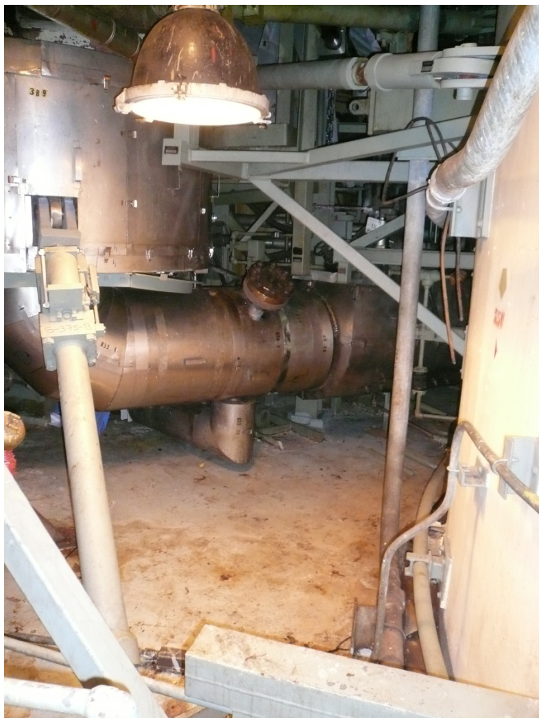
connection at 4" Decon Nozzle RRS
