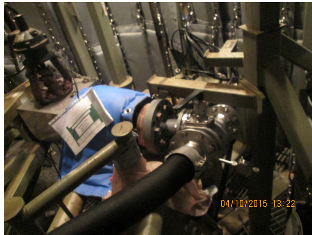
Bottom Drain line connection RWCU
